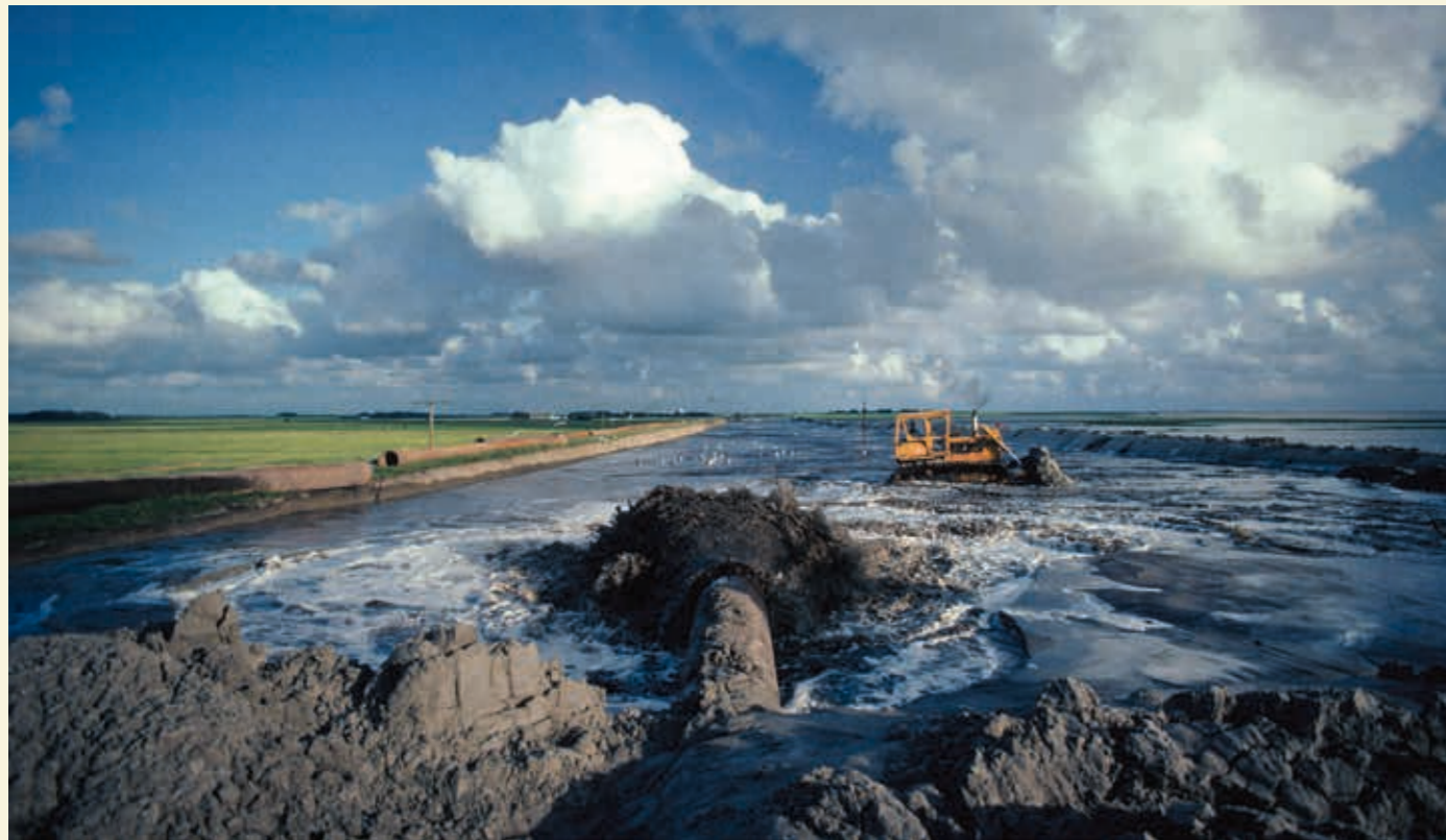
4.8 > In 1985 the Wadden Sea in Schleswig-Holstein was declared a national park. Despite this there was strong criticism to begin with because controversial coastal protection measures were still being carried out, such as the locking of the Nordstrand Bight with a dike formed from sand using hydraulic filling.
