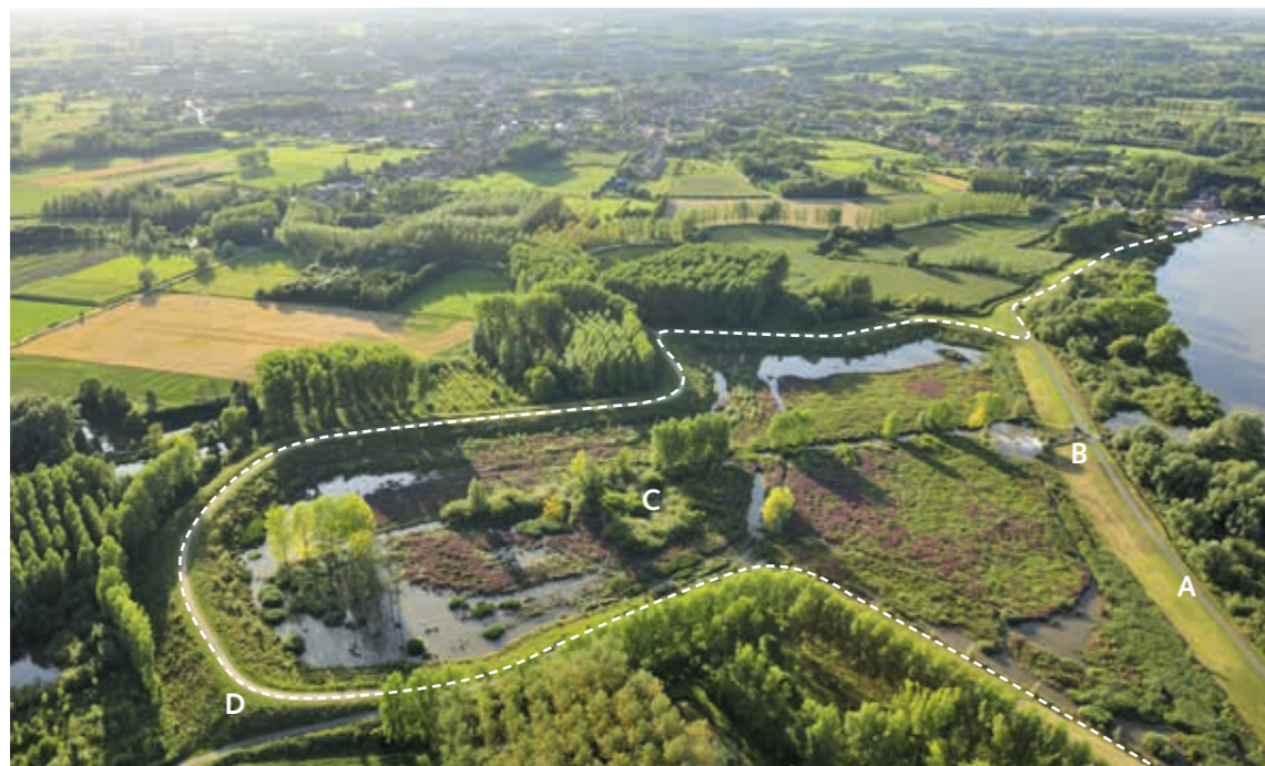
4.20 > New polders are being built on the Scheldt estuary. The existing levee (A) is lowered to function as an overflow dike. The water level within the polder is regulated through a sluice (B) in order to form a wetland area (C). A new ring dike (D), located behind the original location, protects against high water surge.
