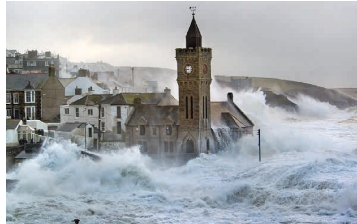
1.22 > The village of Porthleven in the English county of Cornwall is located on an extremely high-energy rocky coast. Accordingly, the shoreline fortifications, including massive walls, are very substantial. Under conditions of very high seas, however, they are hardly noticeable.
